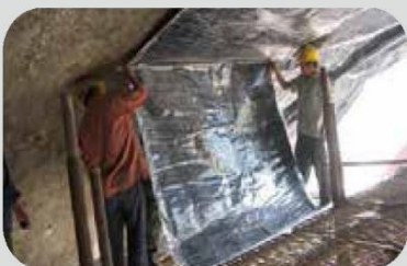
Install the next sheet membrane
