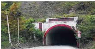
Chongqing Sanpai Mountain Tunnel
