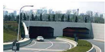
Nanjing Jiuhua Mountain Tunnel
