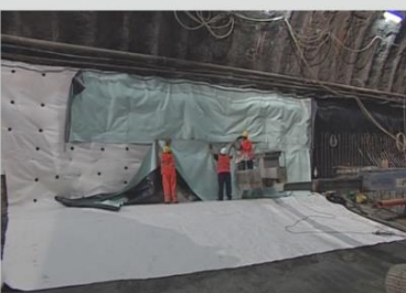
Weld PVC membrane
